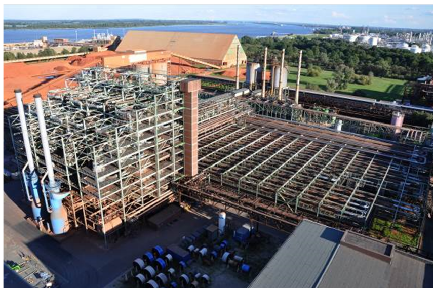
Figure 2. AOS tube digester.
